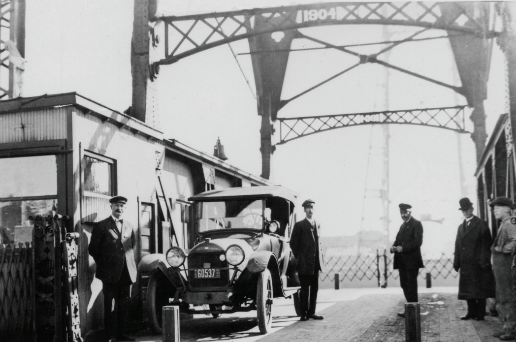
CONDUCTORS AND A FEW PASSENGERS—AND AN AUTOMOBILE—ON THE AERIAL TRANSFER BRIDGE'S GONDOLA CAR, AWAITING MORE PASSENGERS BEFORE CROSSING. BY CREATING ACCESS TO PARK POINT, THE BRIDGE MADE MINNESOTA POINT EVEN MORE POPULAR. ADD TO THAT A DRAMATIC INCREASE IN AUTOMOBILE TRAFFIC IN DULUTH FROM 1901 TO 1925, AND THE BRIDGE WAS RENDERED INADEQUATE BY THE MID 1920S.
