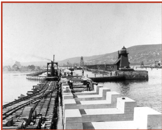
L to R: The process of building the concrete piers of the Duluth Ship Canal and a few of the thousands of men who helped built them between 1896 and 1902. [IMAGES: LSMC]
