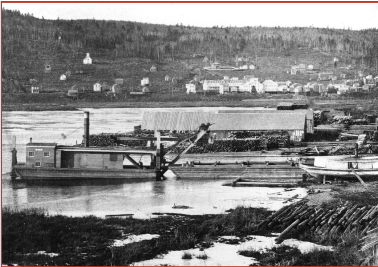
The dredging tug Ishpeming cutting the Duluth Ship Canal in 1870 with the developing new city of Duluth in the background. [IMAGE: LSMC]
