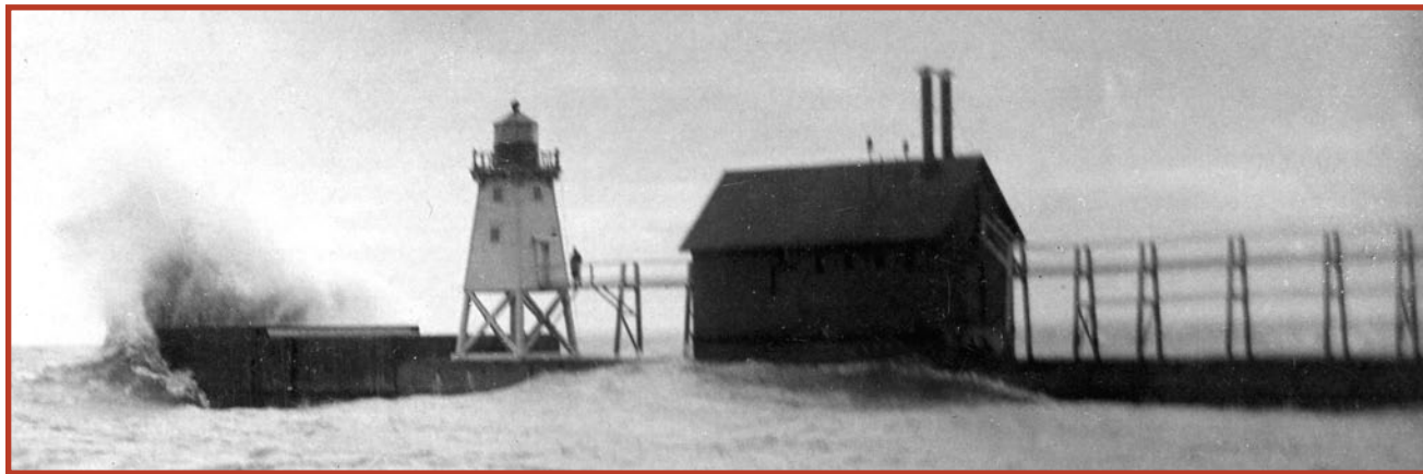
The original South Breakwater Light and keeper's house. Note the raised walkway, built to help keeper's reach the light during storms. [IMAGES: LSMC]
