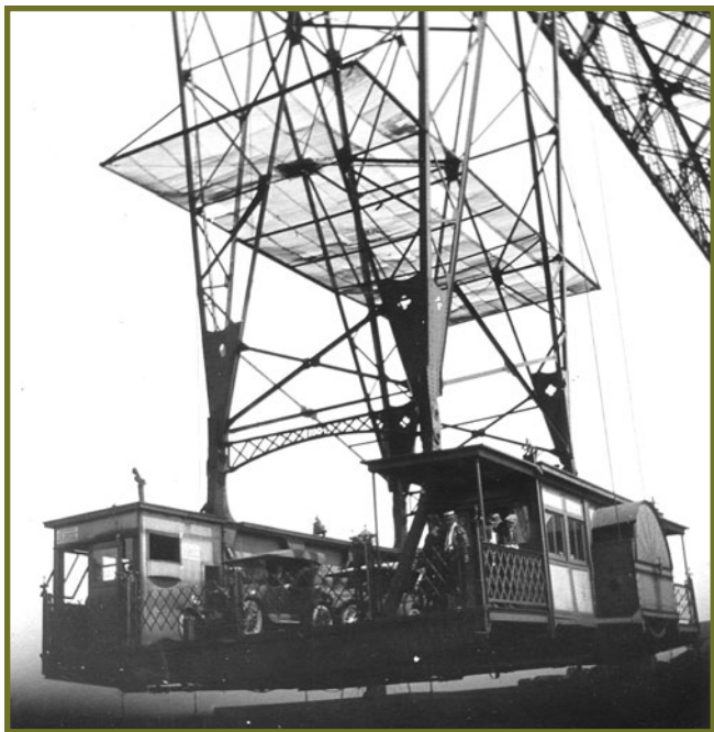
The gondola car showing the ice shield installed in 1906. [IMAGE: LSMC]
