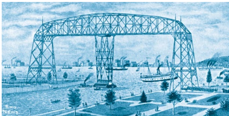
This drawing of Cap Turner’s plans appeared in Engineer News magazine in 1901.[IMAGE: JJHL]
