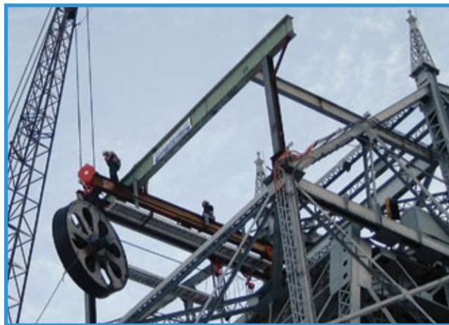
Workers replace a sheave in 1999. [IMAGE: DSN]
