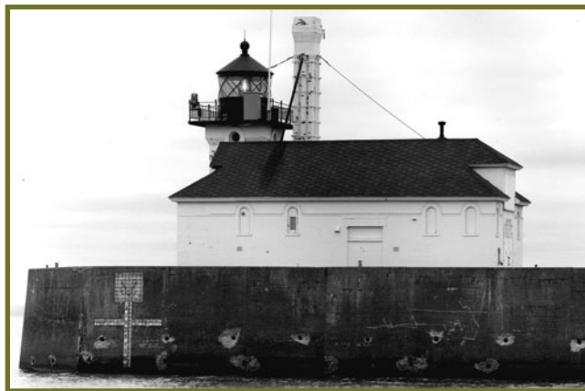
Gaillard's wave-level indicator tiles on the canal's south pier, photographed in 1985 by Grandmaison Studios. [IMAGE: LoC]
